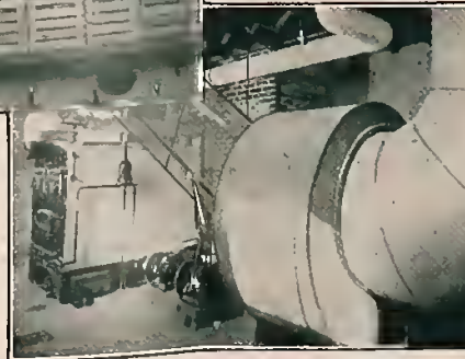
Directly below is shown the automatic oil heating plant; also the mammoth fan and piping. At the extreme right the air intake and steam-heated radiators which heat the air drawn in by the fan.
